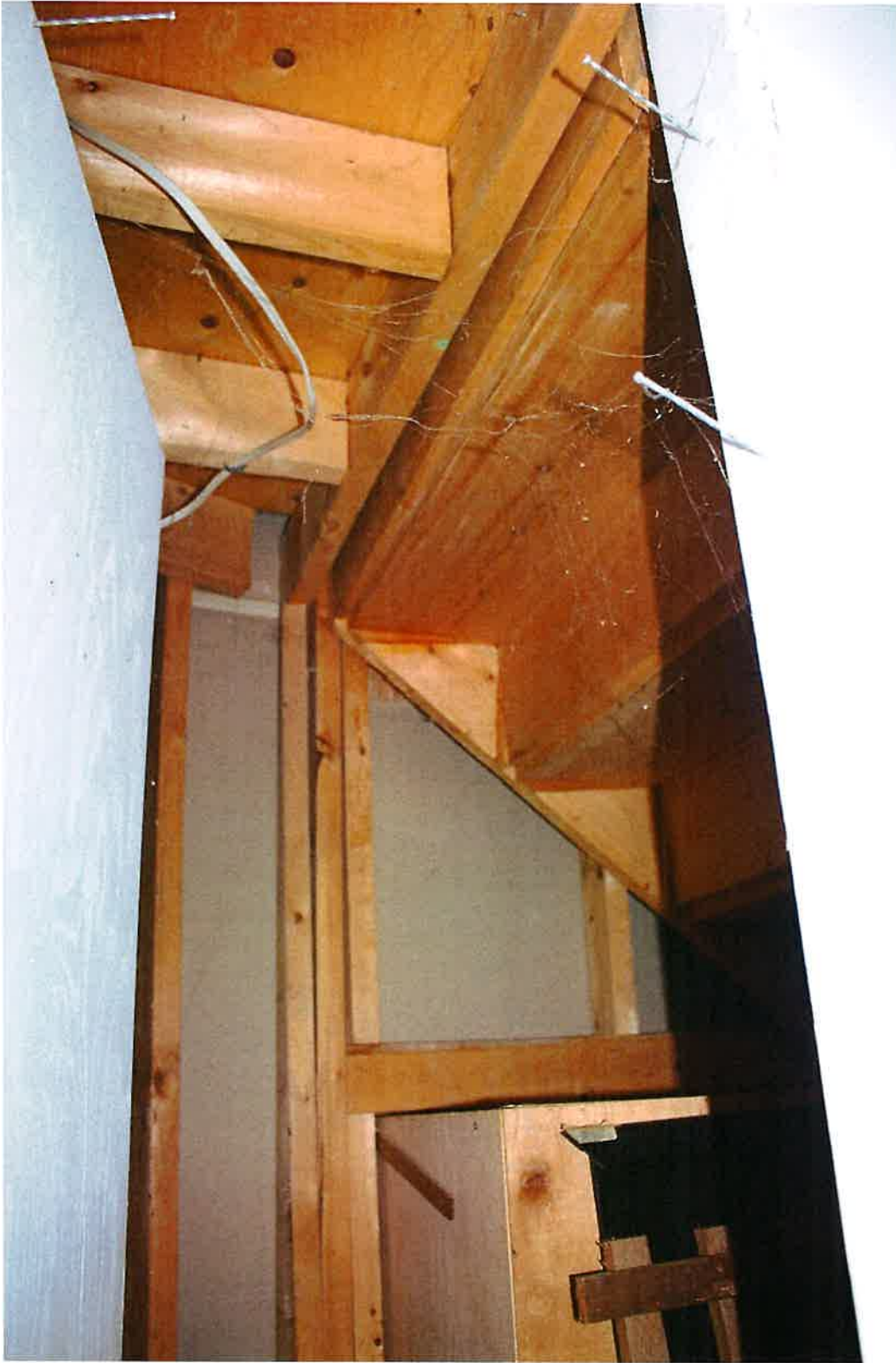
Figure 1: Underside of rear staircase showing new woodwork.
