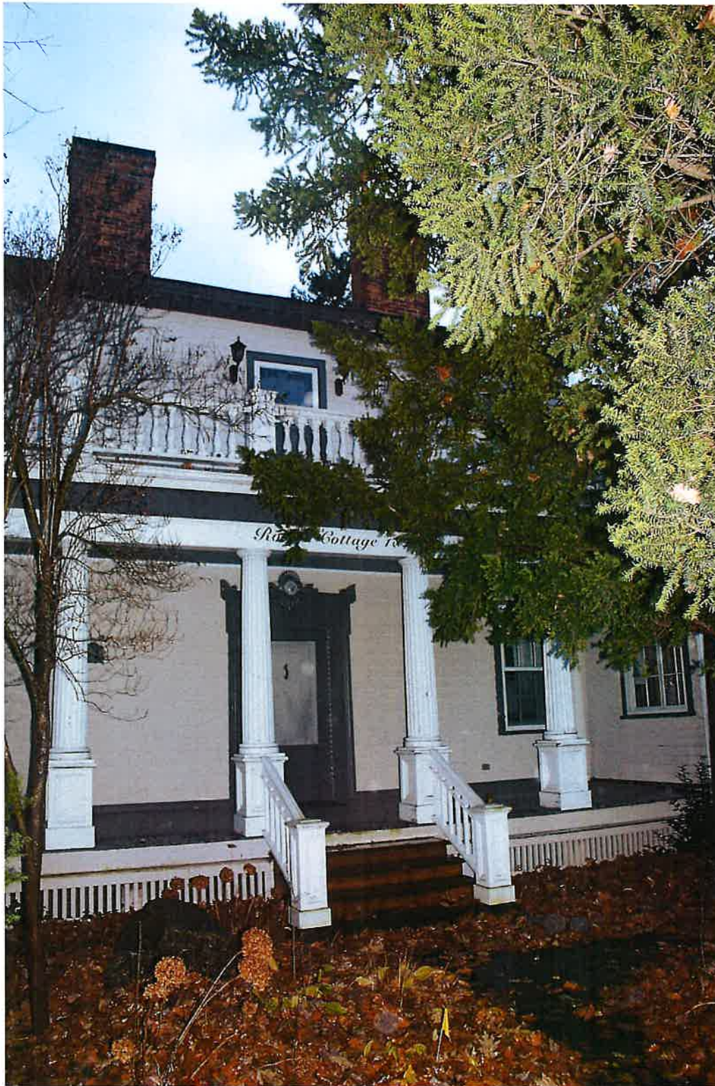
View of 187 Queen Street from the east looking towards the main entrance.
