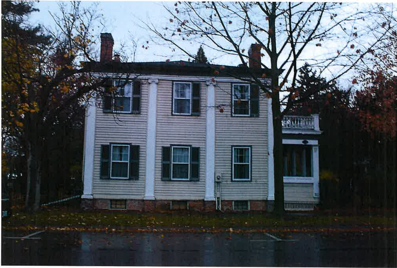
View of 187 Queen Street from Queen Street looking towards the southern elevation.
