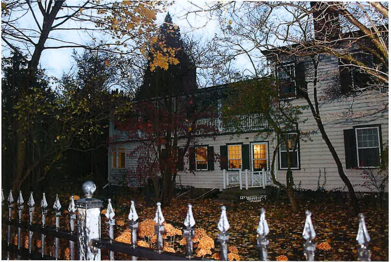
View of 187 Queen Street from the west looking towards the western elevation.
