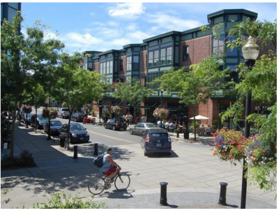
Multi-storey mixed-use buildings with activity at the ground level
